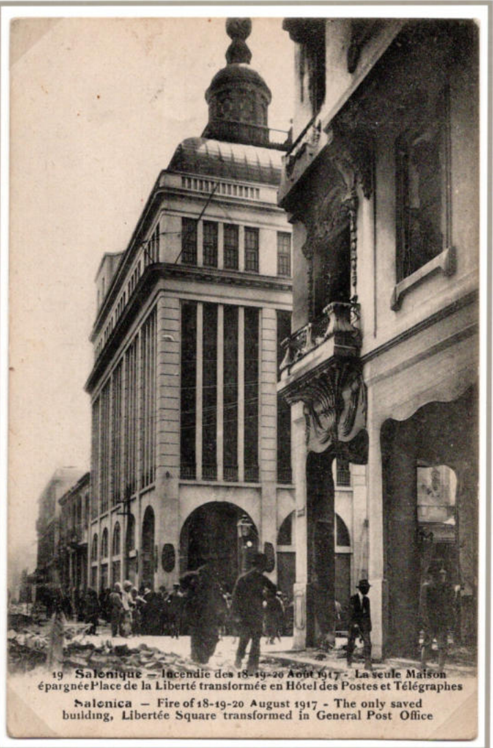
Central Post Office from 1917 to 1930, on Liberty Square.
